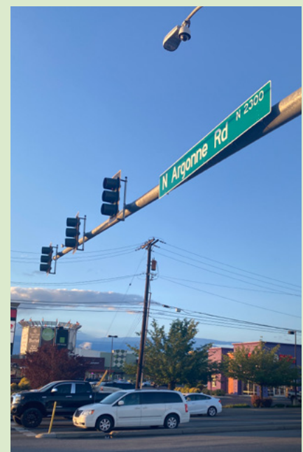
Camera located at the N Argonne Road intersection in Spokane, WA that provides real-time data for traffic signal timing updates.
