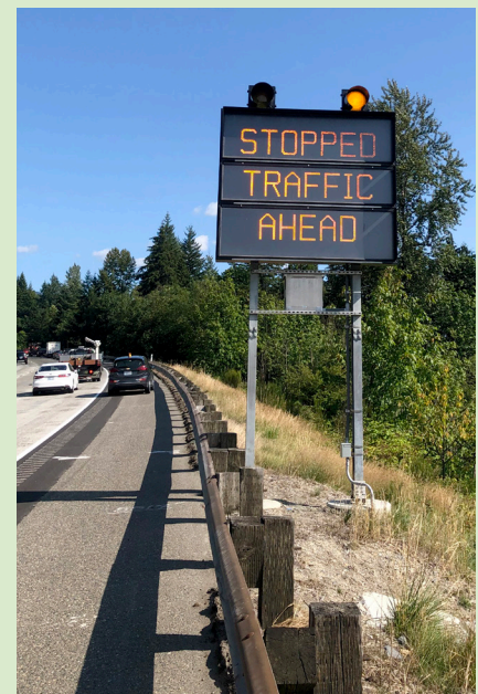
A variable message sign on the side of a freeway displays the message “Stopped Traffic Ahead” and attached beacons flash orange lights.
